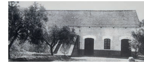
The building housed the cold storage chamber.
