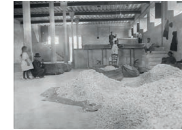
Image of the stifling facility viewed from the marked point
